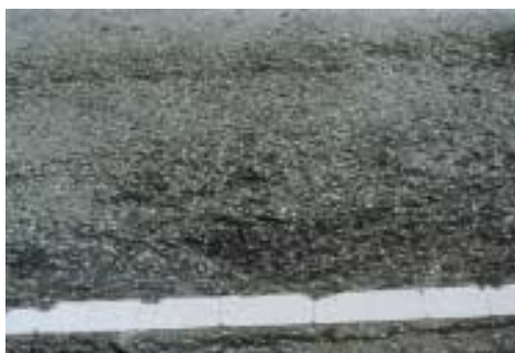
Figura A.20 – desgaste (SHRP, 2003)
