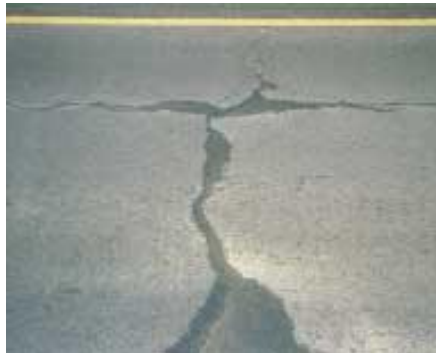
Figura A.22 – Bombeamento (SHRP, 2003)
